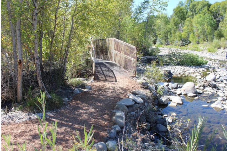
Photo 3: Severely eroded bank viewed northwest toward the bridge. This section of trail just off the bridge experiences flooding and erosion during Spring runoff, and a major piece was eroded with Spring 2019's high runoff.
