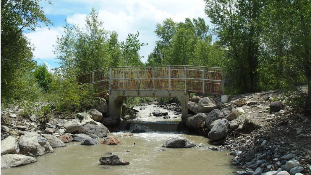
Photo 1: Current primitive bridge over Minnesota Creek during low flow summer months
