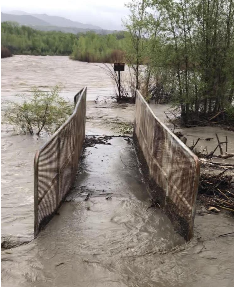
Photos 4 & 5: Bridge and Confluence of Minnesota Creek and the North Fork of the Gunnison. Flooding during Spring Runoff (bottom photo) jeopardizes the stability of the river bank and bridge.
