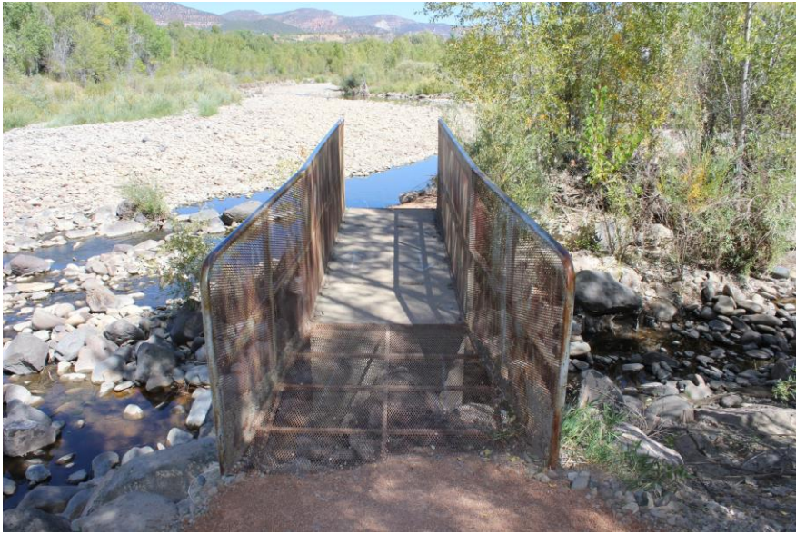
Photo 3: Severely eroded bank viewed northwest toward the bridge. This section of trail just off the bridge experiences flooding and erosion during Spring runoff, and a major piece was eroded with Spring 2019's high runoff.
